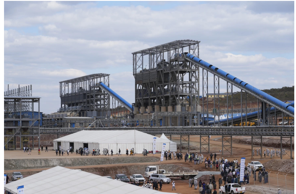
Prospect Lithium Zimbabwe's processing plant in Goromonzi about 80 miles southeast of the capital Harara which was officially commissioned in July 2023
