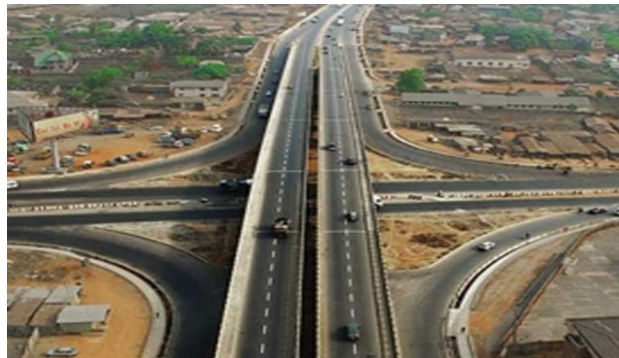
Insufficient houses and infrastructure
